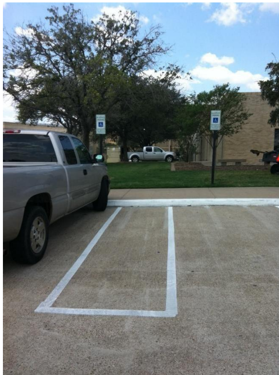
Parking Area 74 - No Compliant Curb Ramp
