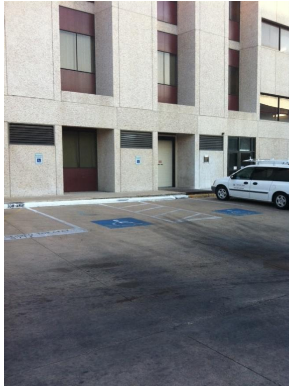
Parking Area 57 - No Compliant Curb Ramp
