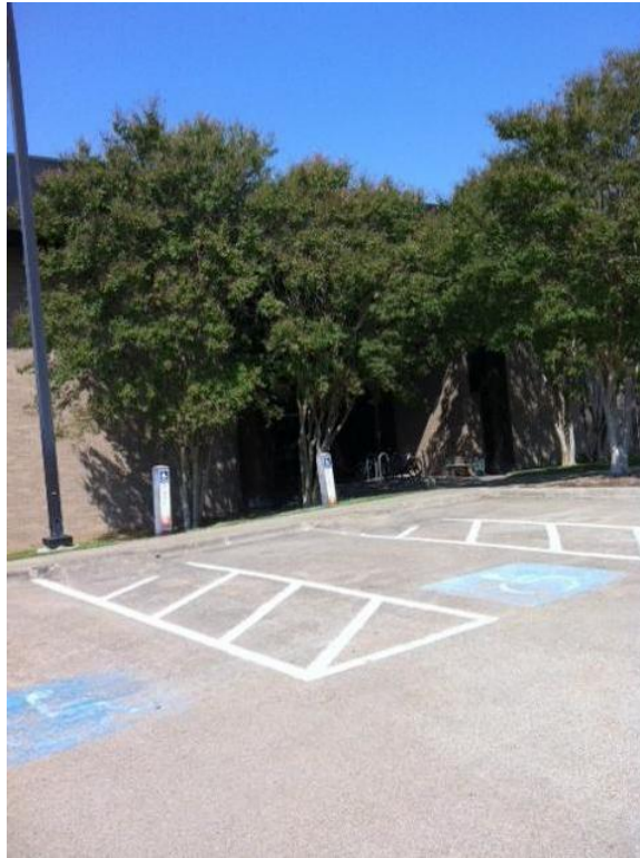
Parking Area 108 – No Compliant Curb Ramp and Non Compliant Signage
