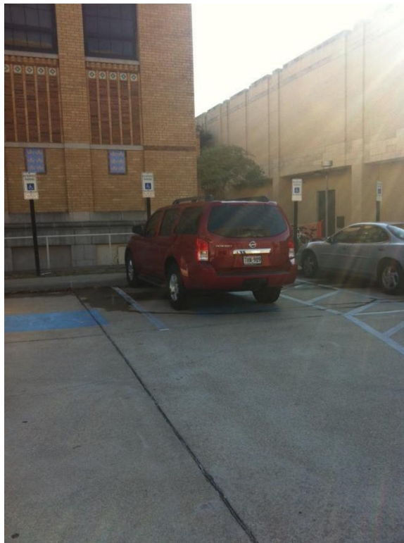
Parking Area Spence Street - No Compliant Curb Ramp and No Accessible Aisle
