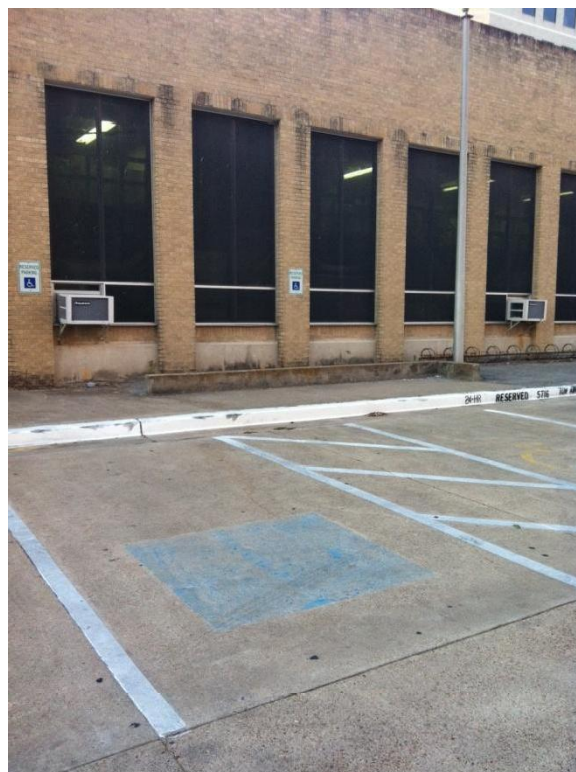
Parking Area 57 - No Compliant Curb Ramp
