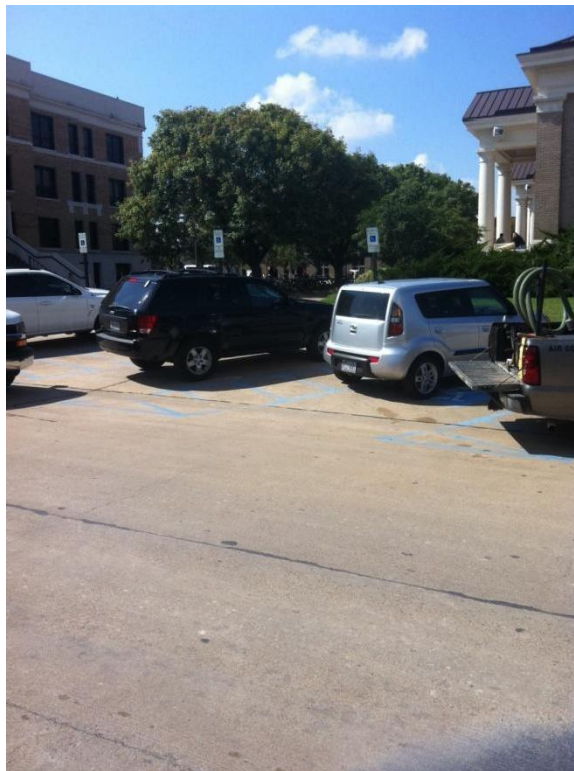
Parking Area Asbury Street – No Compliant Curb Ramp and Running Slope Exceeds 1:48
