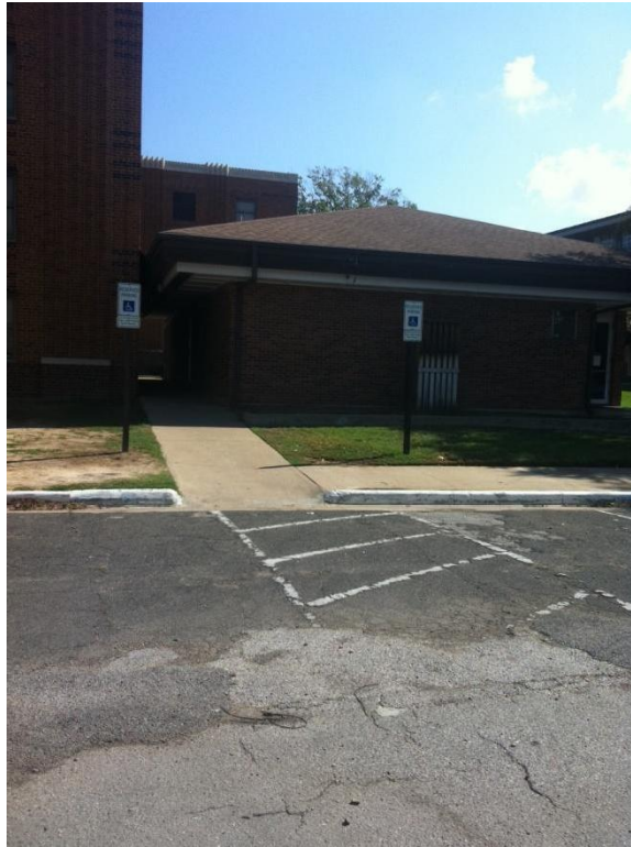
Parking Area 30c - Non Compliant Curb Ramp
