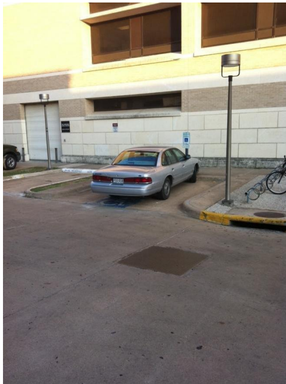
Parking Area 14 – No Compliant Curb Ramp, No Accessible Aisle and Running Slope Exceeds 1:48
