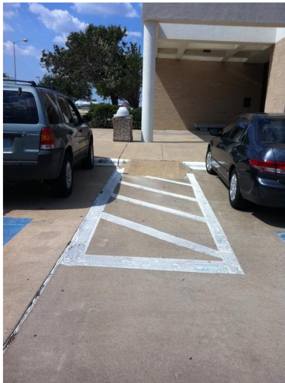
Parking Area 85 - Non Compliant Curb Ramp
