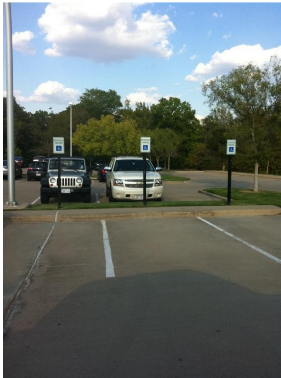
Parking Area 111 - No Compliant Curb Ramp and No Accessible Aisles
