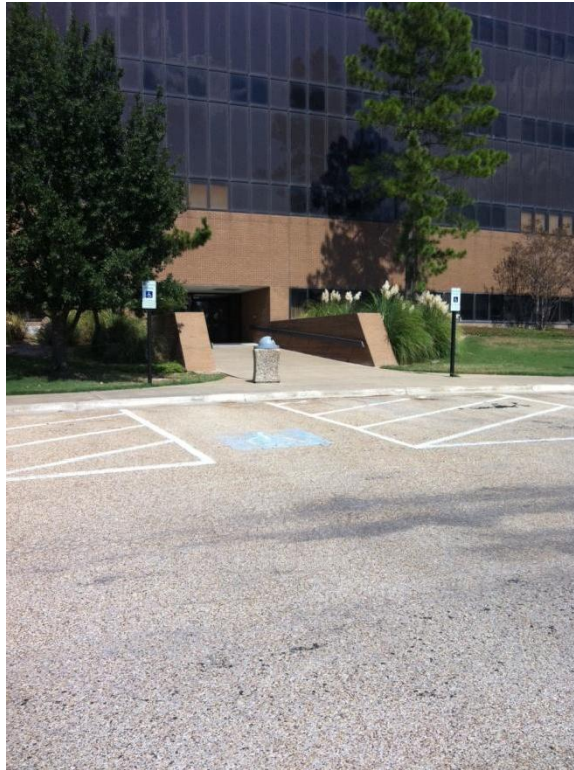
Parking Area 73 - No Compliant Curb Ramp
