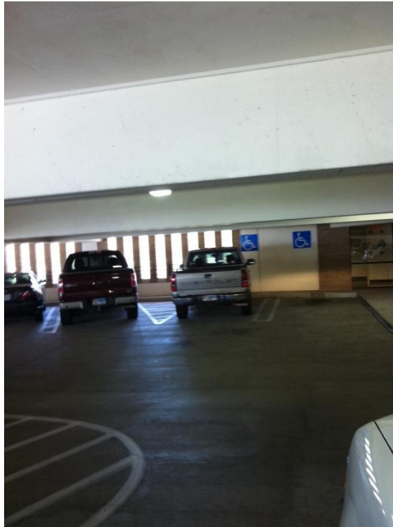
Parking Area University Center Parking Garage - No Compliant Curb Ramp and No Accessible Aisles
