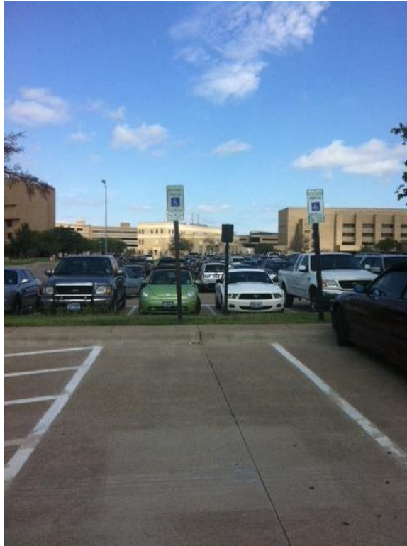
Parking Area 74 – No Compliant Curb Ramps
