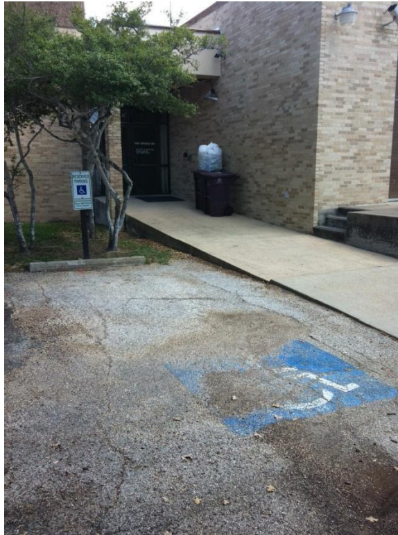
Parking Area 59 - No Compliant Curb Ramp and No Accessible Aisle
