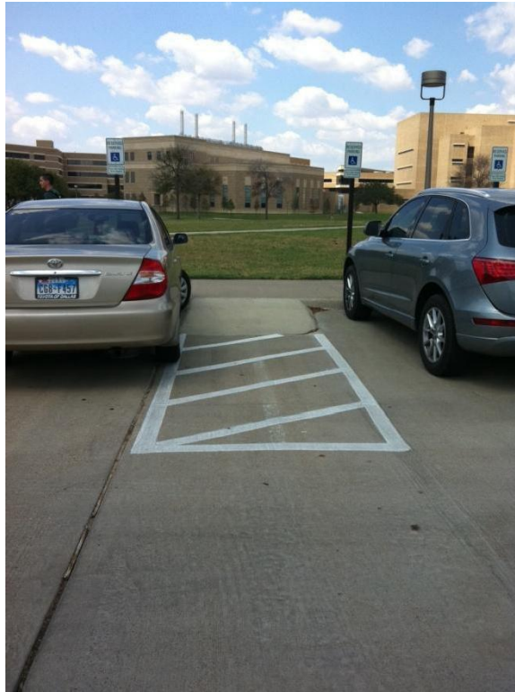
Parking Area 74 - Non Compliant Curb Ramp
