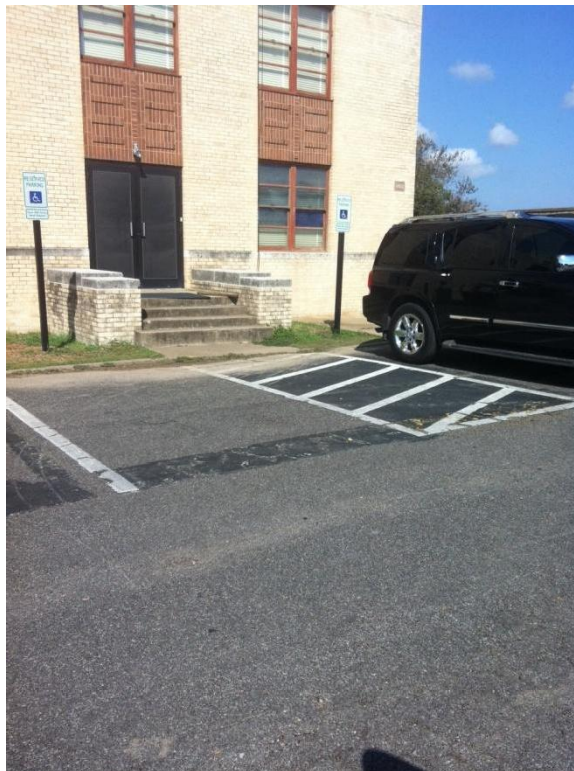
Parking Area 77 - No Compliant Curb Ramp
