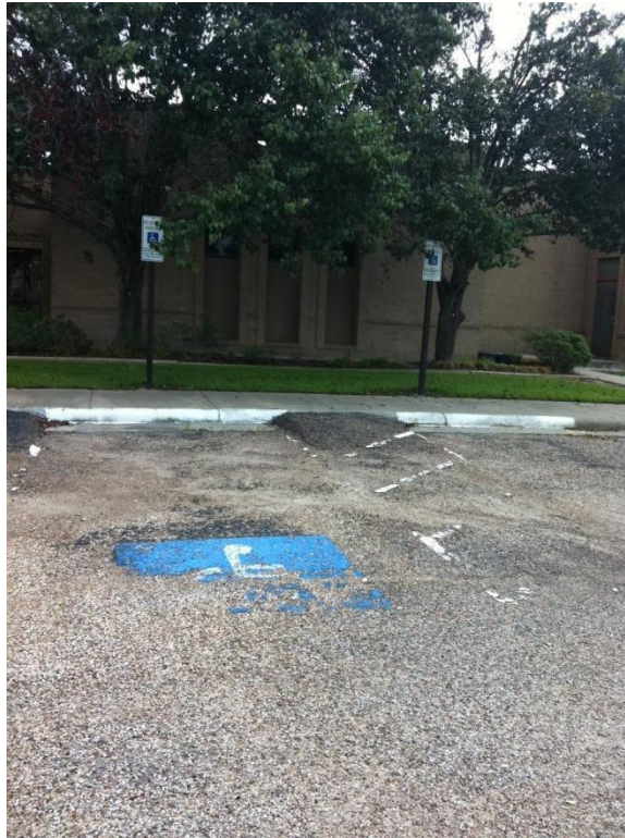
Parking Area 37 - Non Compliant Curb Ramps
