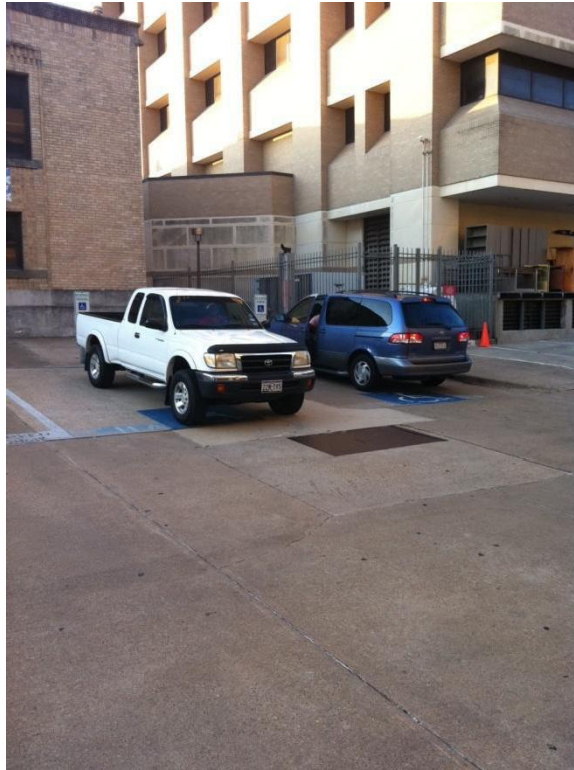
Parking Area 14 – No Accessible Aisles and Running Slope Exceeds 1:48
